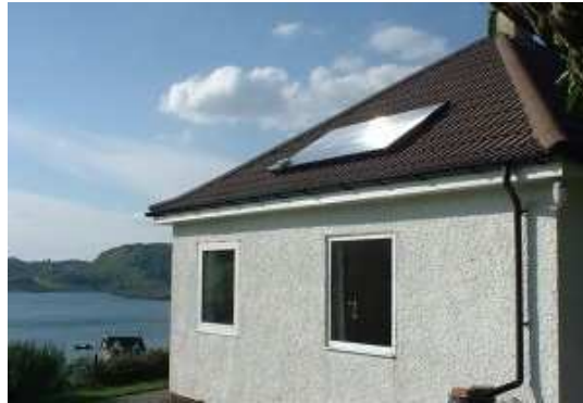
Solar Panels – this is one of a range of innovative energy efficiency measures across Argyll & Bute which also contribute towards tackling fuel poverty.
